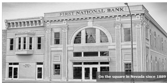
Figure 3. Exterior of the First National Bank, Nevada, Missouri as restored in 1999.
